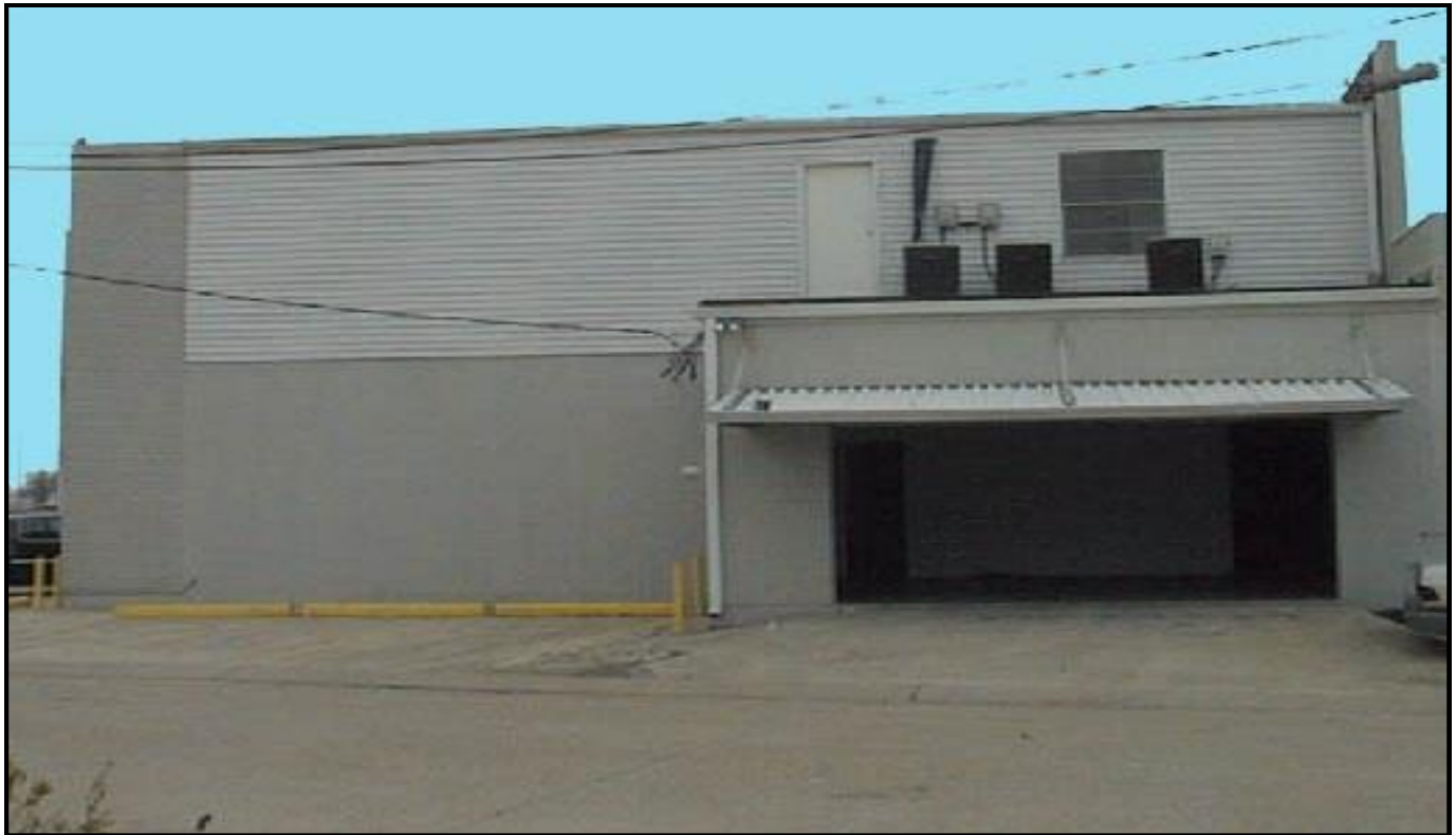
Warehouse Exterior Access
